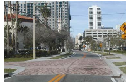
Speed table Photo courtesy of FHWA.
