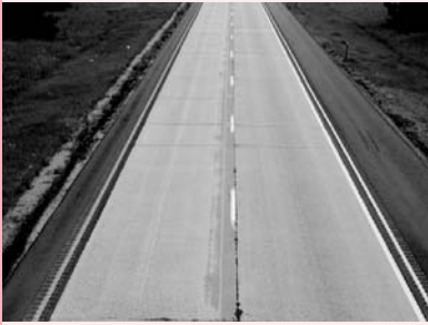
An edge line on the road, a parallel line in the rumble strip.
