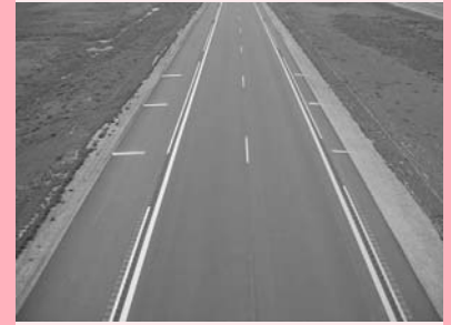
An edge line on the road, a parallel dashed line in the rumble strip.
